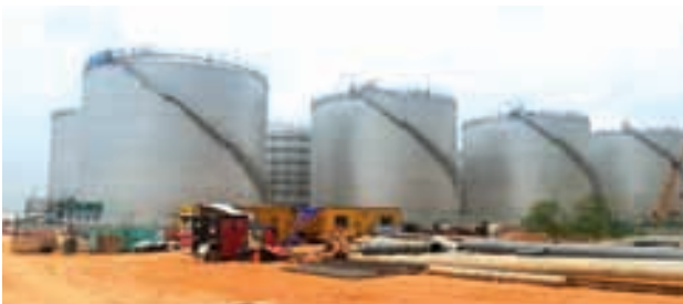
Project Reference: Bitumen Tank In Pasir Gudang using ALCOM's aluminium sheet
