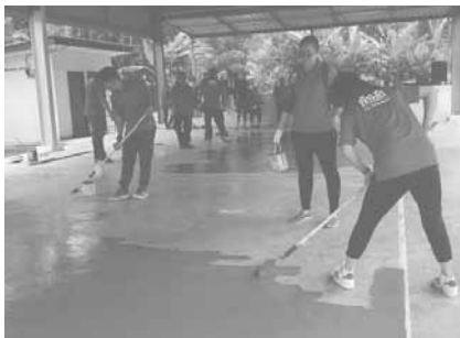
Upgrading the open hall
