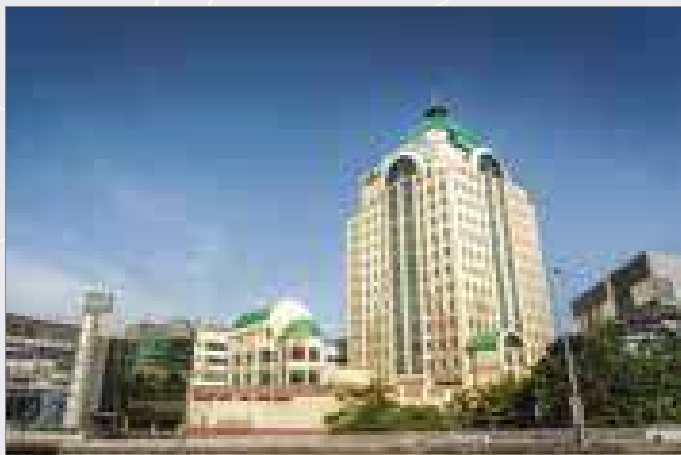
7 Menara Axis ◀ Office
