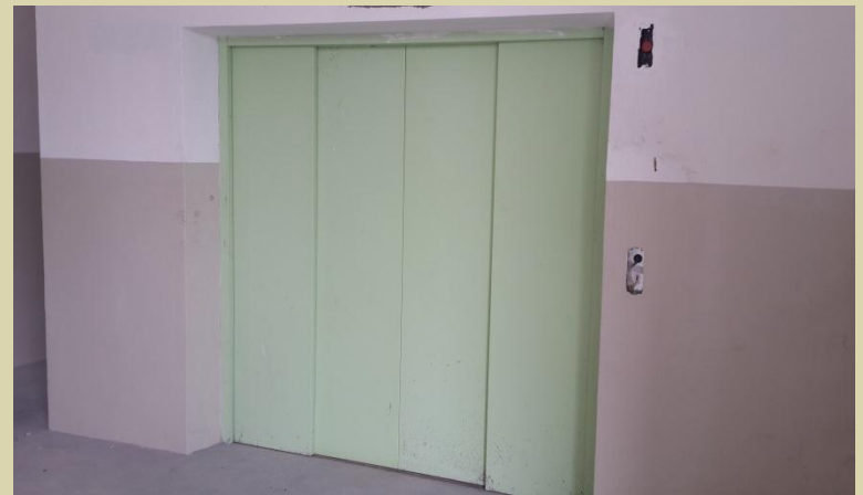
New Cargo Lift
