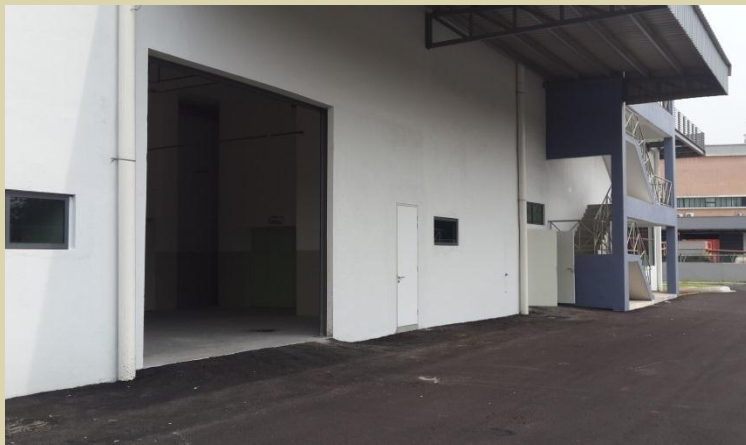
Cargo Loading Bay
