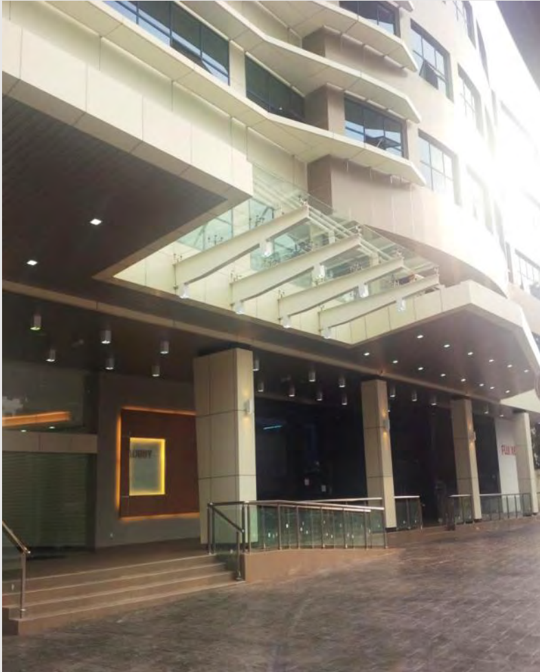
Drop-off lobby with disabled ramp
