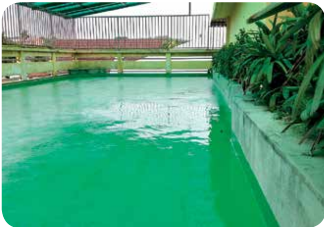
Coated the rooftop concrete slab with epoxy paint to reduce heat absorption.
