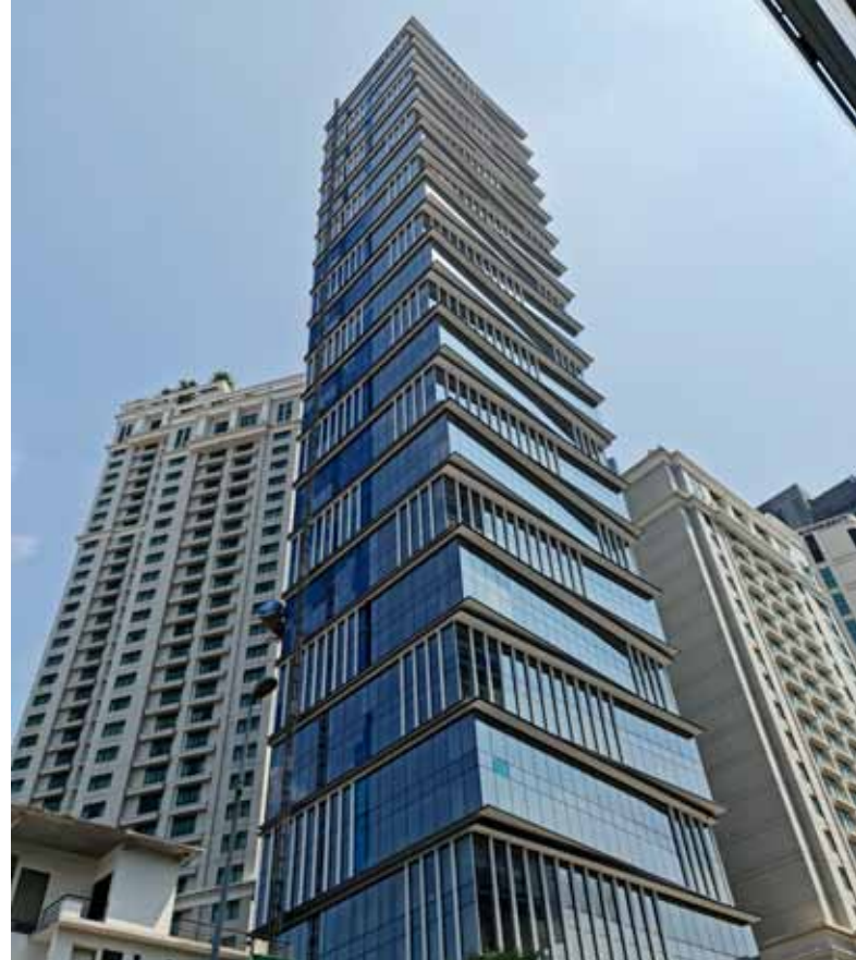
Capri Hotel, Jalan Imbi (Construction)
