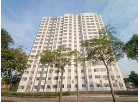
Rumah Selangorku, Subang Bestari (Construction)
