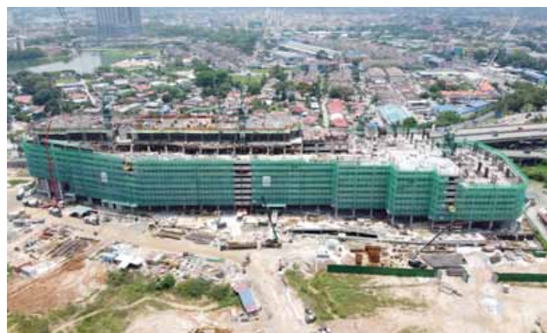
99 Residence Development, KL North (Construction)
