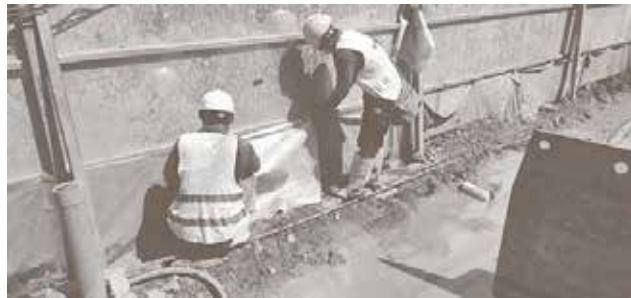
Erosion and sediment control measures in project site in Cambodia (Slope protection and silt fence).
