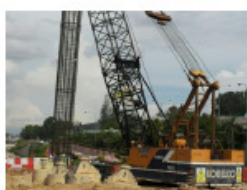
Bored Piling: Klang Valley MRT Package V6
