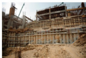
Bored Piling: Jalan Medang Serai, Bangsar high-end apartments
