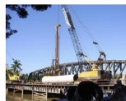
Bored Piling: Ipoh-Padang Besar double-tracking
