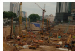
Bored Piling: Pavilion KL shopping centre
