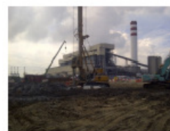
Bored Piling: Tanjung Bin Power Plant
