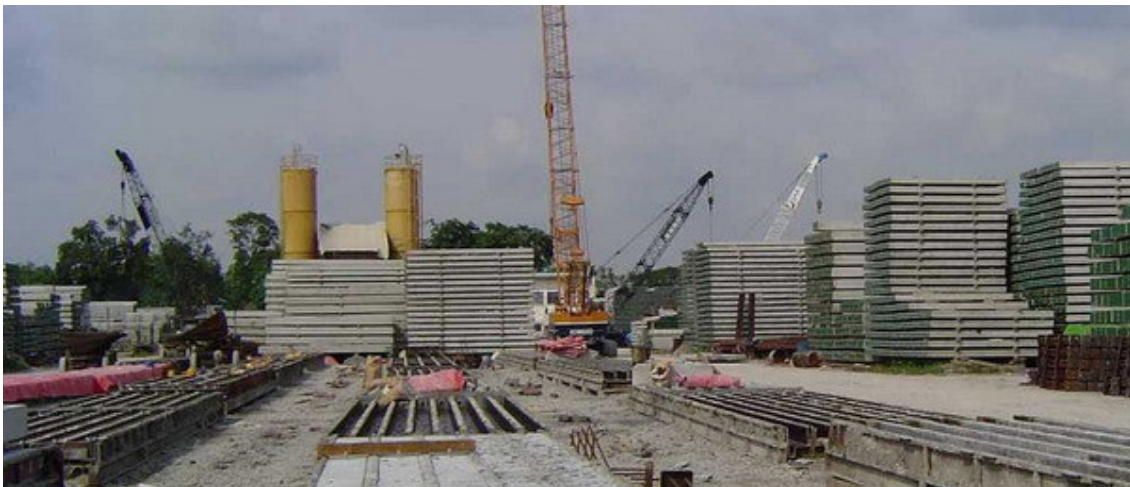
ECIC's precast yard at Kranji
