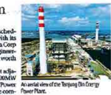
An aerial view of the Tanjung Bin Energy Power Plant.
