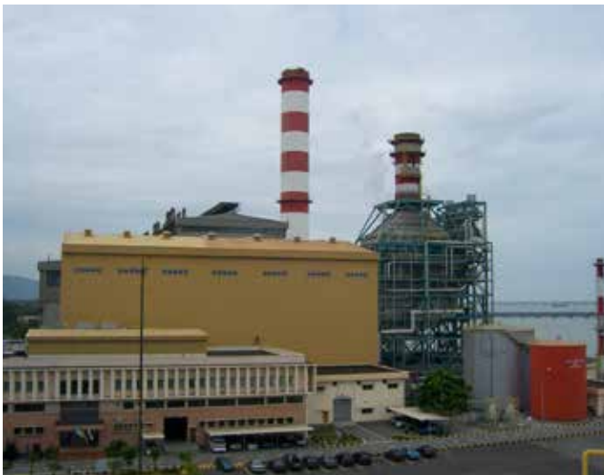
Prai Power Plant, Penang
