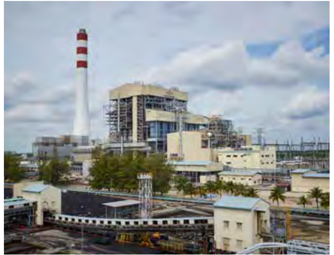
Tanjung Bin Energy Power Plant, Johor
