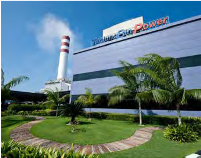
Tanjung Bin Power Plant, Johor
