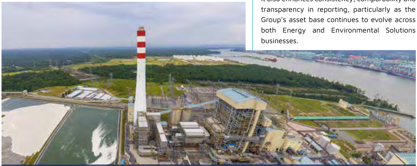
Contributing to a balanced energy mix, Tanjung Bin Energy Power Plant emphasises operational efficiency and dependable base load generation.
