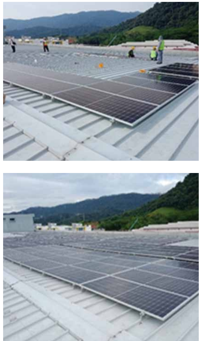
Figure 2: Installation of solar PV system on rooftop of manufacturing facility
