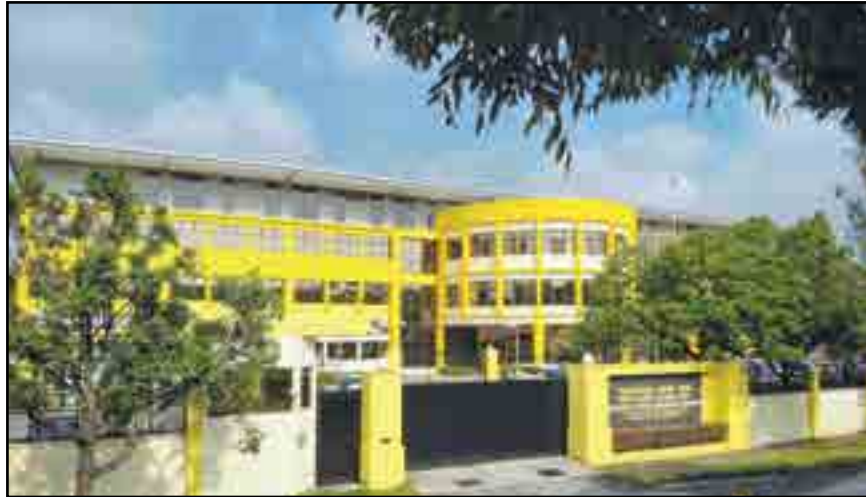
Poh Kong Jewellery Manufacturer Sdn. Bhd. in Shah Alam constructed an additional floor to the building.
