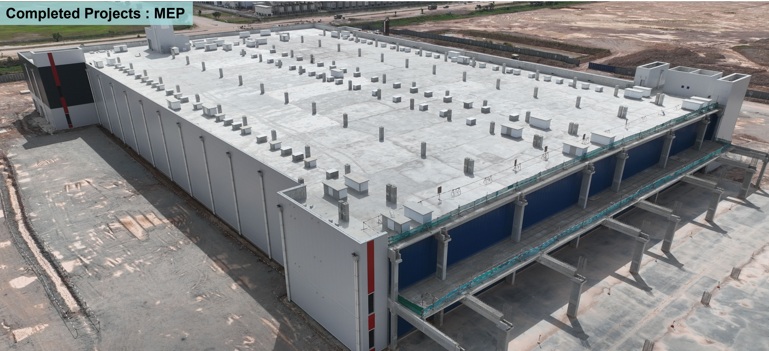
Data Centre at Sedenak, Johor
