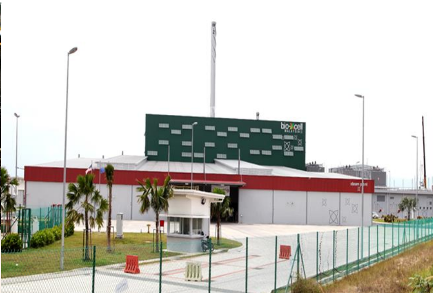
Central Utilities Facilities
