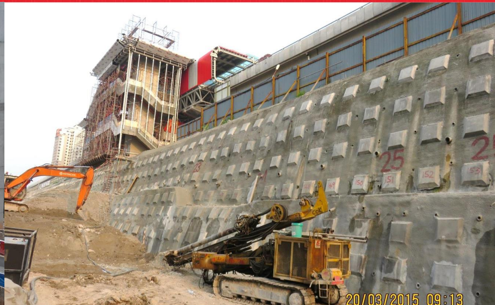
Earth Retaining System
