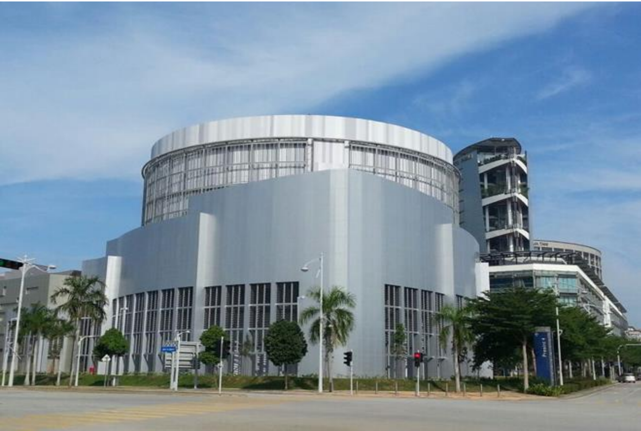
Gas District Cooling Plant - Putrajaya
