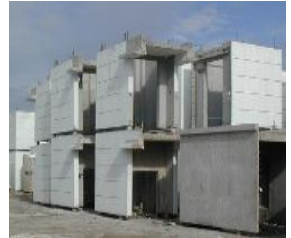
Lift Core Wall
