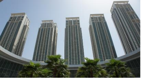
Al-Reem Island Phase 1, Plot 1 Completed : 2009 USD362mil
