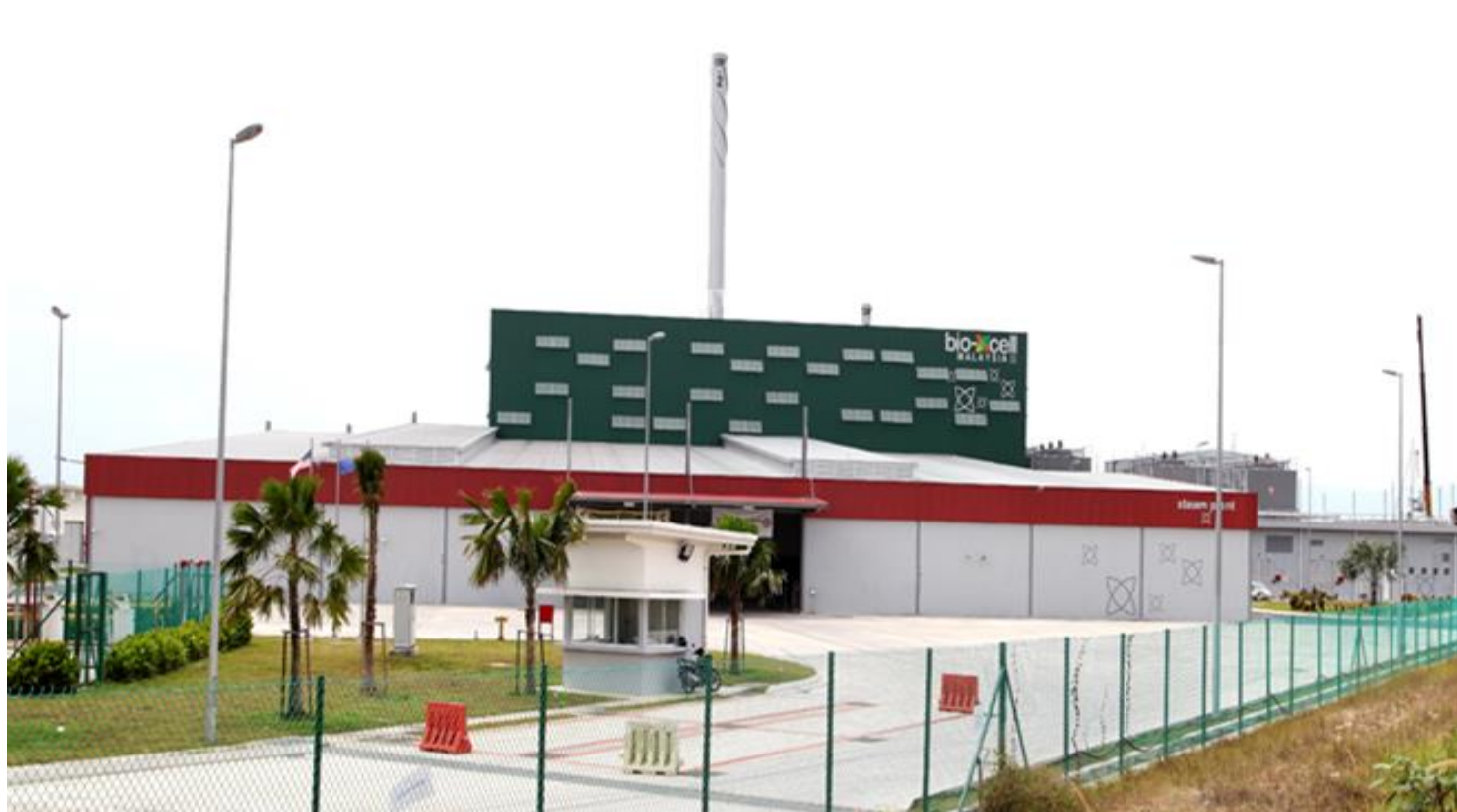
Central Utilities Facilities
