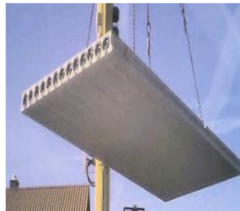
Hollow Core Slab
