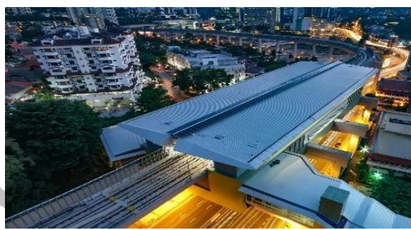
MRT Package V4, Klang Valley Completed : 2016 RM1,172mil
