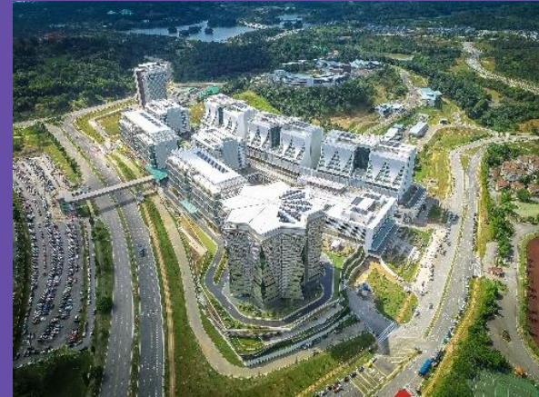
Building Construction Services
