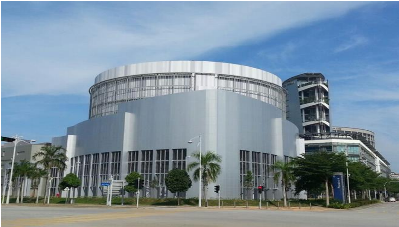
Gas District Cooling Plant – Putrajaya
