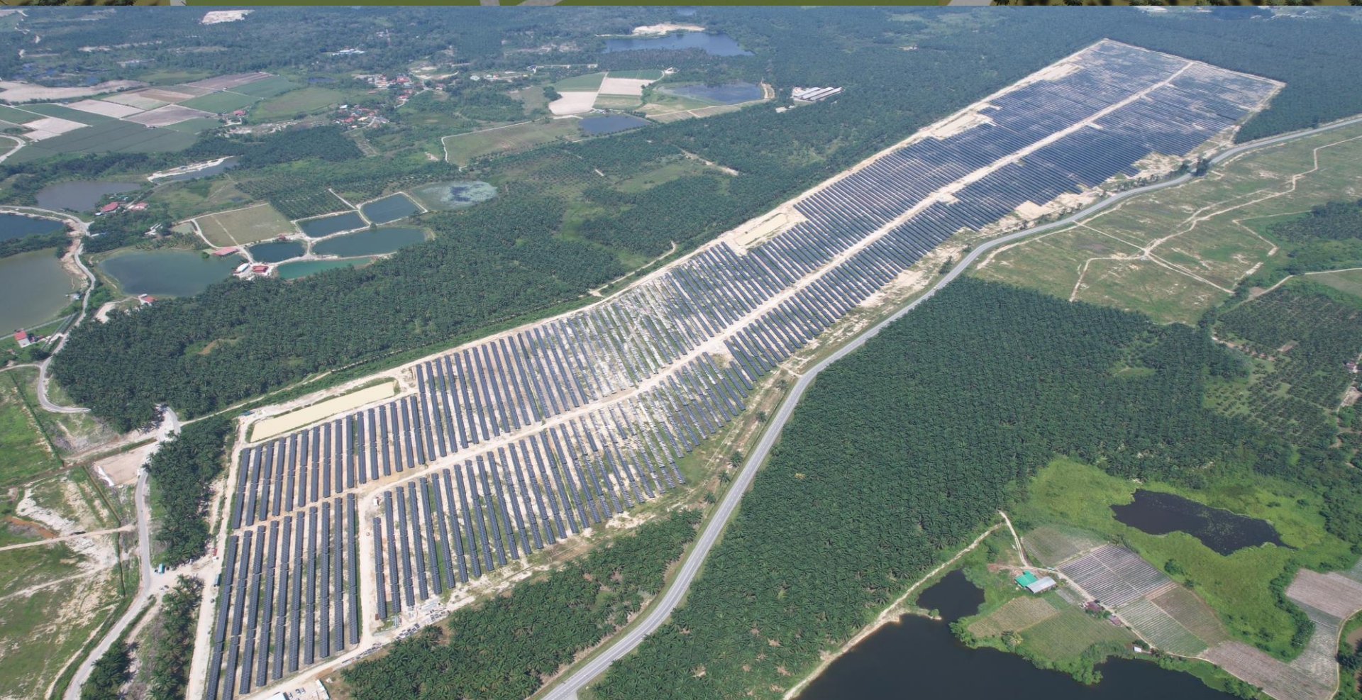
Large Scale Solar 4, Gopeng, Perak (50MW)
