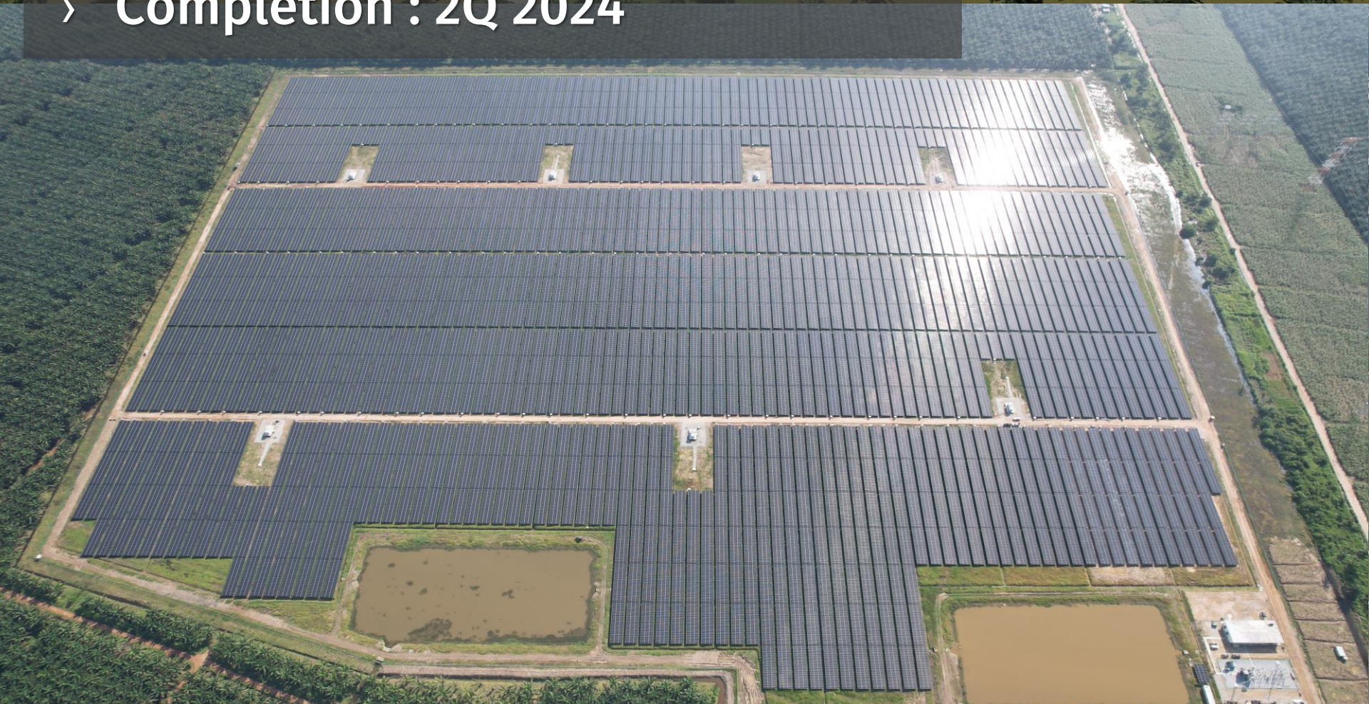
Large Scale Solar 4, Kapar, Klang (50MW)
