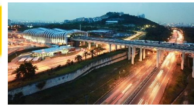
LRT Package B Completed : 2015 RM569mil
