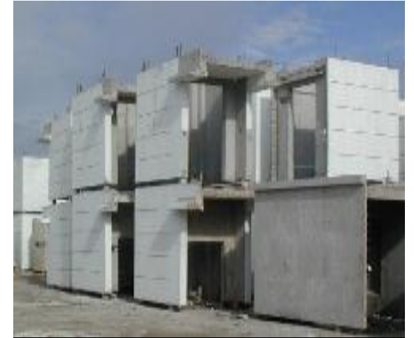
Lift Core Wall
