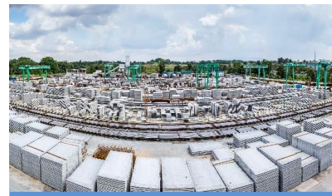
Manufacturing and Sale of Precast Concrete Products
