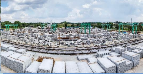
Manufacturing and Sale of Precast Concrete Products
