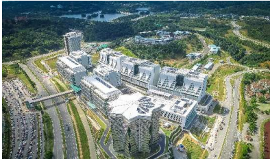
Building Construction Services
