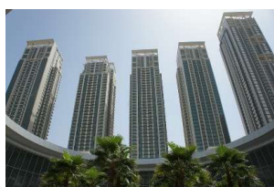
Al-Reem Island Phase 1, Plot 1 Completed : 2009 USD362mil
