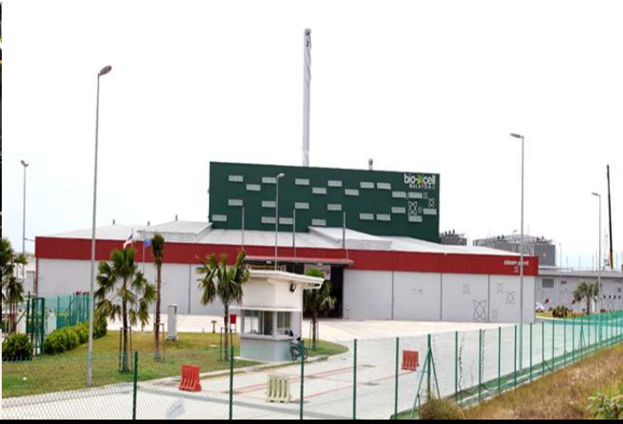
Central Utilities Facilities
