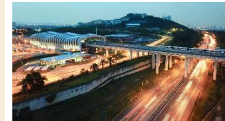
LRT Package B Completed : 2015 RM569mil
