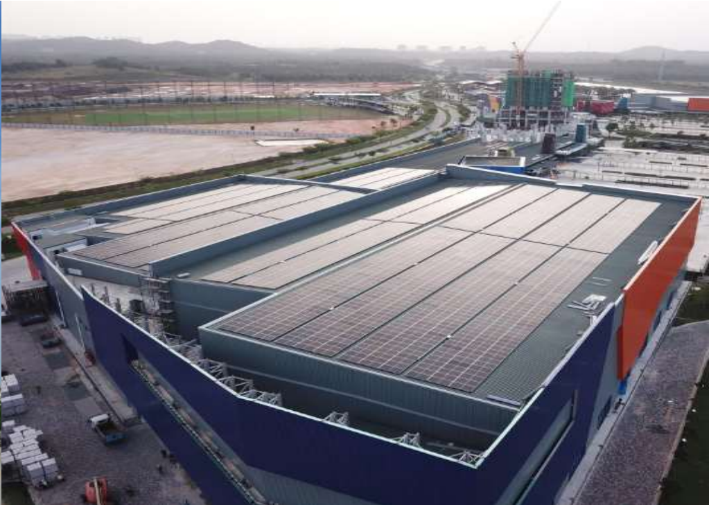
Roof Top Solar – Sunway Iskandar
