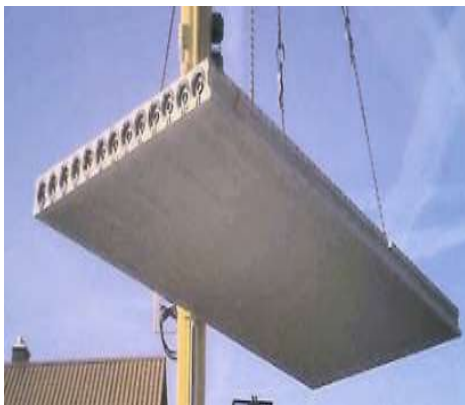
Hollow Core Slab
