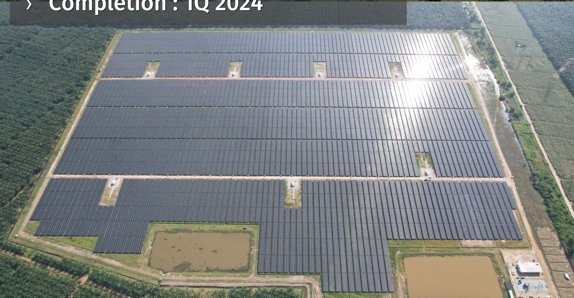
Large Scale Solar 4, Kapar, Klang (50MW)
