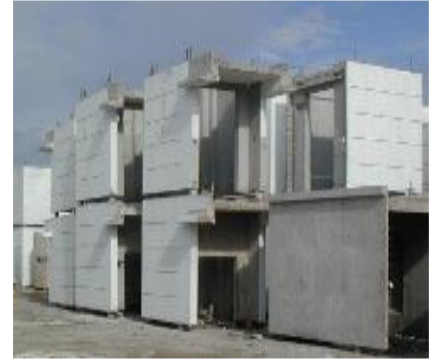
Lift Core Wall
