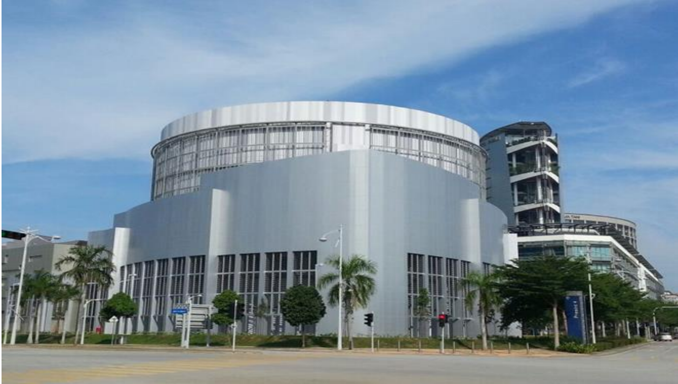
Gas District Cooling Plant - Putrajaya
