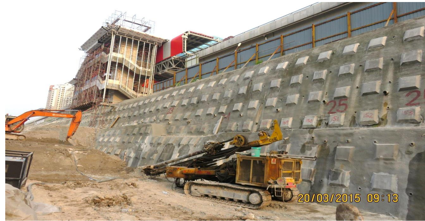
Earth Retaining System
