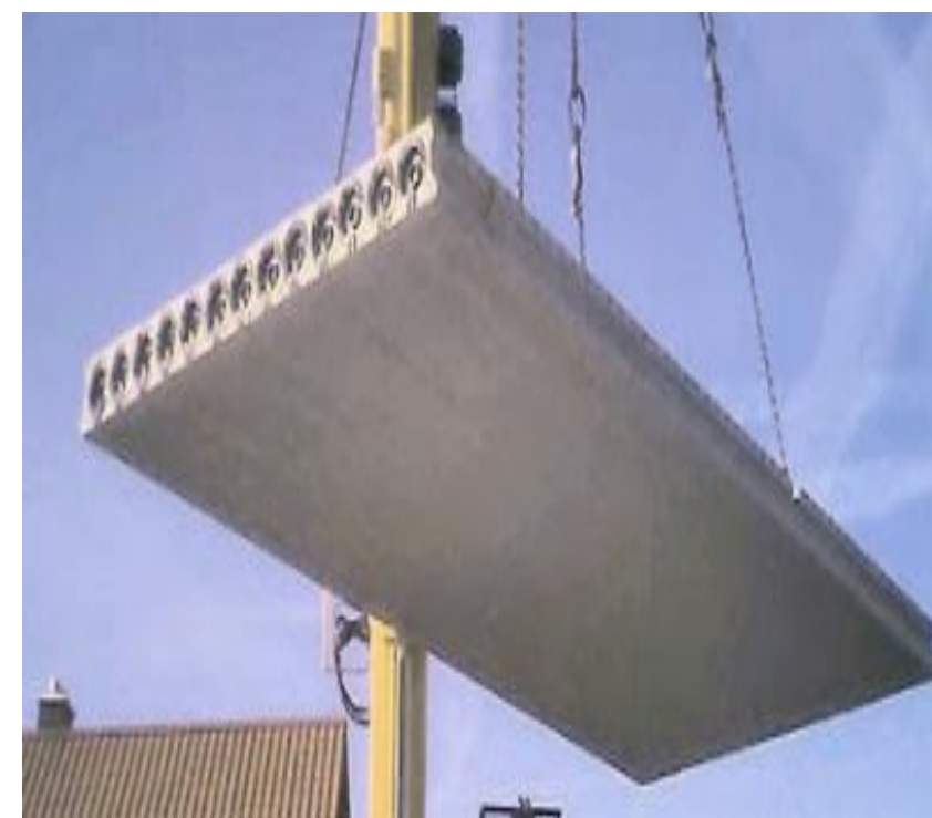
Hollow Core Slab
