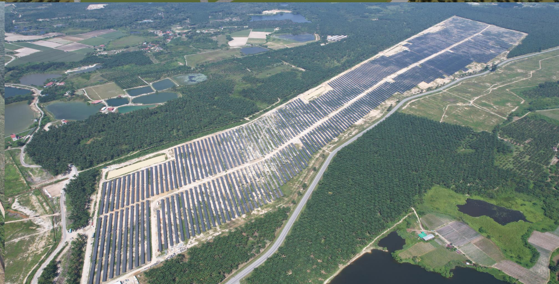
Large Scale Solar 4, Gopeng, Perak (50MW)
