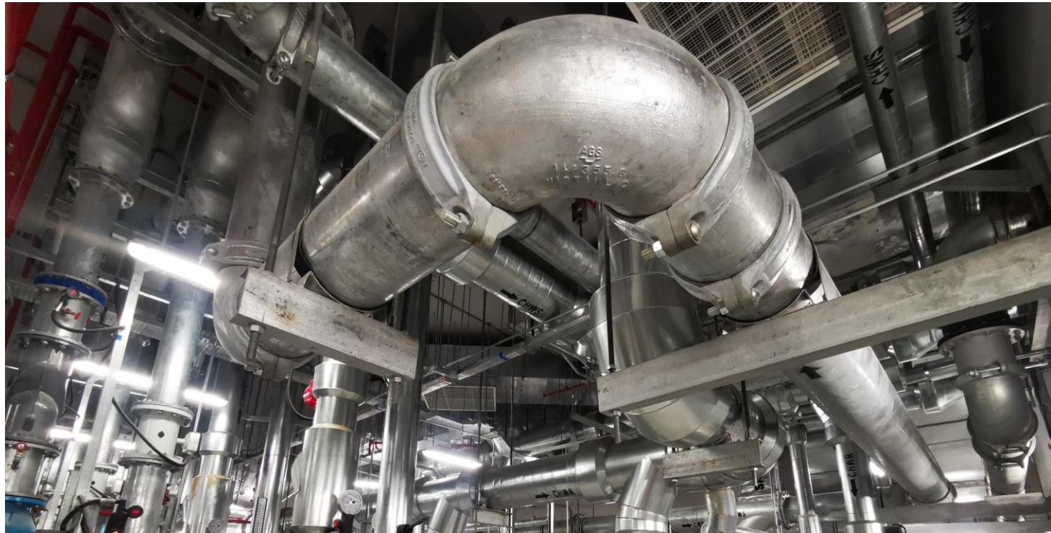
MRT Sentul West Underground Station
