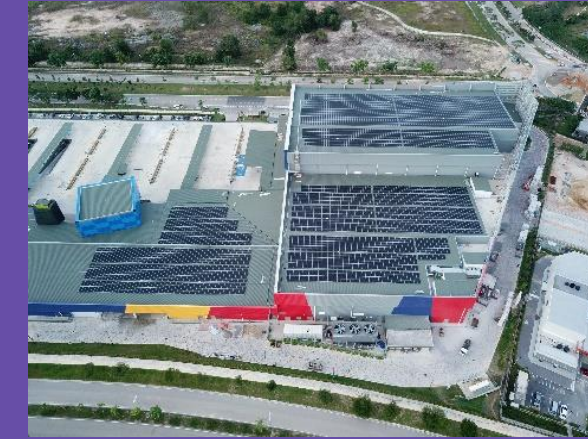
Sustainable Energy Services
