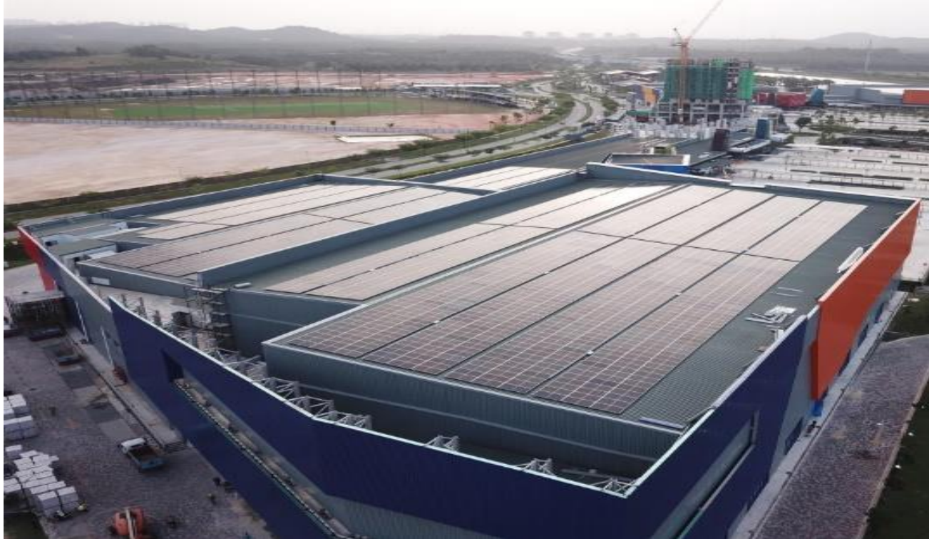
Roof Top Solar – Sunway Iskandar
