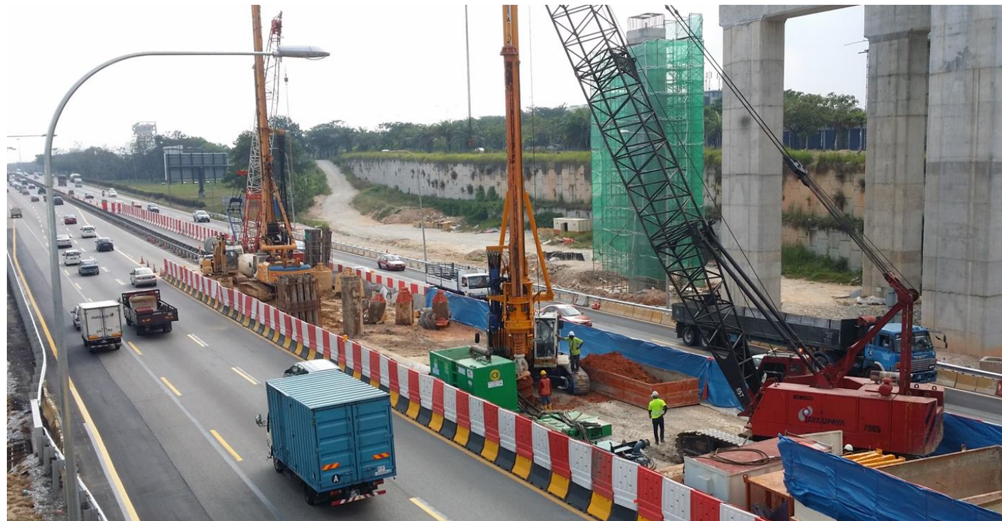
Pile Foundation Works
