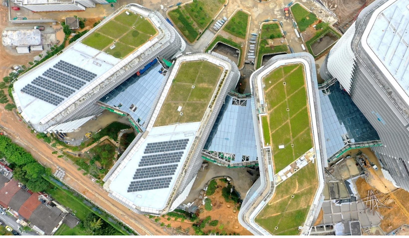
TNB HQ Campus Phase 2 – KL
