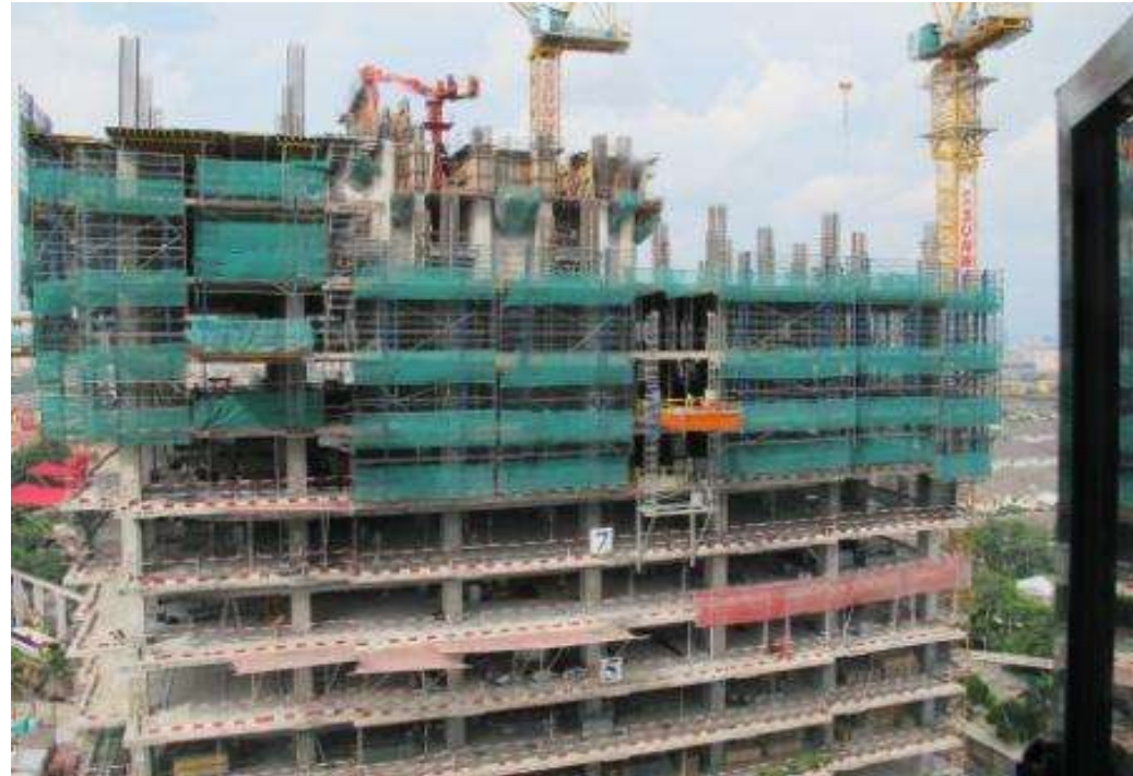
Construction progress photo taken at actual site on 8 Jan 2013
