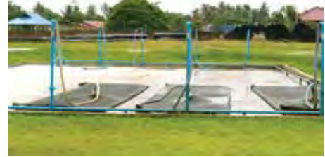
Water treatment plant residual management system using GeoTube® Dewatering Containers
