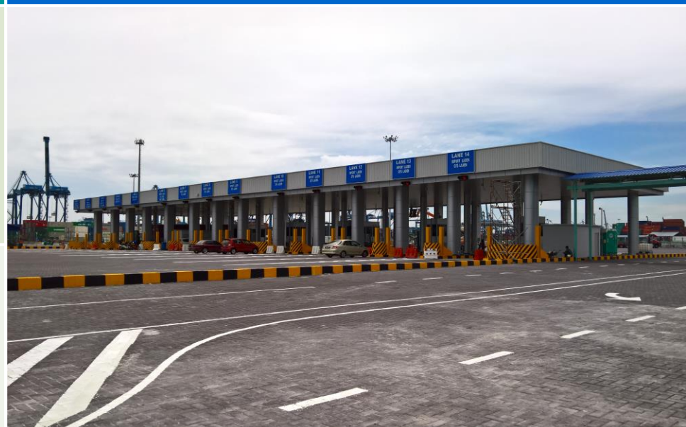
The 2 nd container terminal gate is being completed with 14 lanes for exiting haulier trucks
