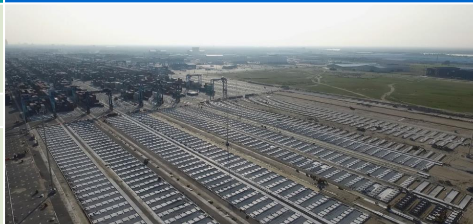
CT8 Container Yard Zone W and Zone X near completion
