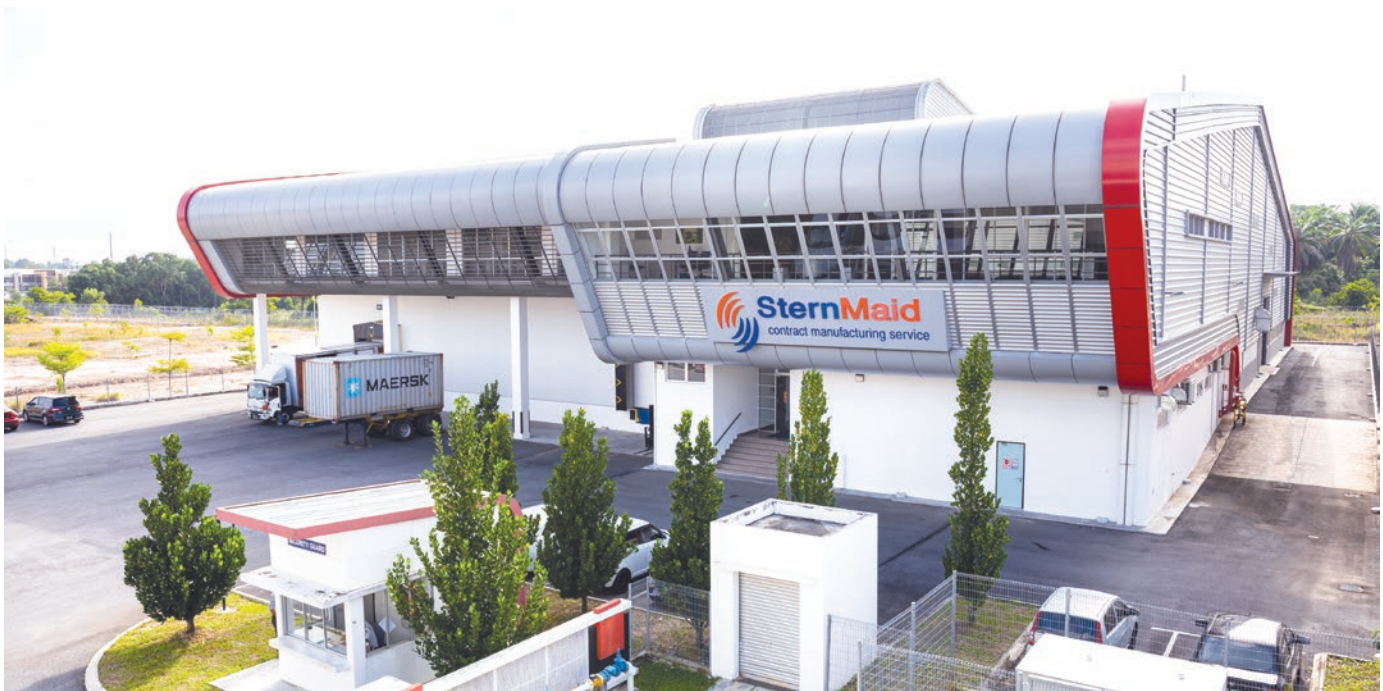
Nusajaya Tech Park Facility 2
