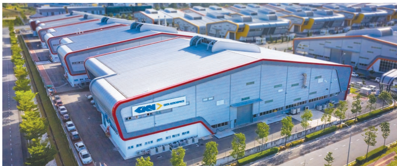
Nusajaya Tech Park Facility 1
