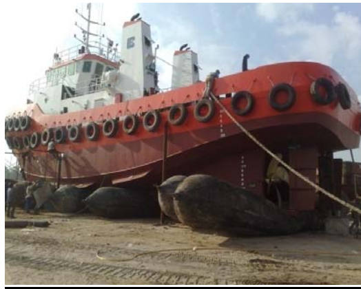
Building of 2400 HP Twin Screw Steel Tug Boat – OCEANLINE 281, 282, 283 and 285
