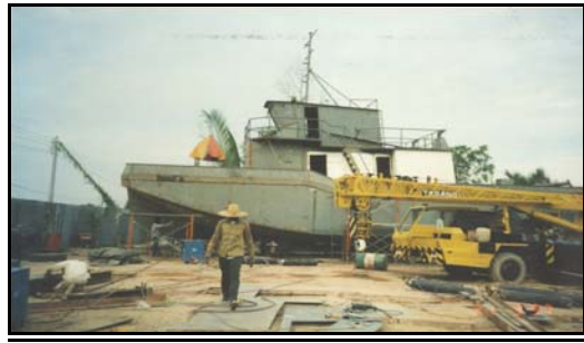
Building of 800HP Anchor Handling Tug 'CATHAY 8' - Year Built 1997
