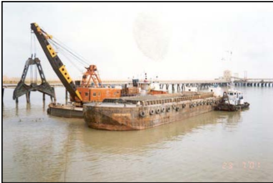
PICTURE 3: CLAMSHELL DREDGER (5 NOS)
