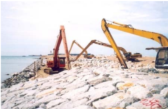
PICTURE 2: ROCK REVETMENT
