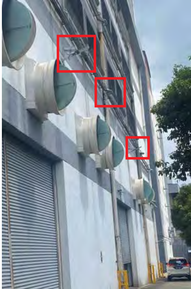
Solar street lightings installed at factory perimeters
