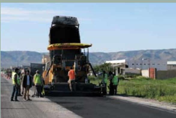
Road rehabilitation work in Libya
