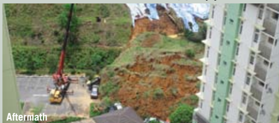
The 2007 landslide incident at Precint 9, Putrajaya
