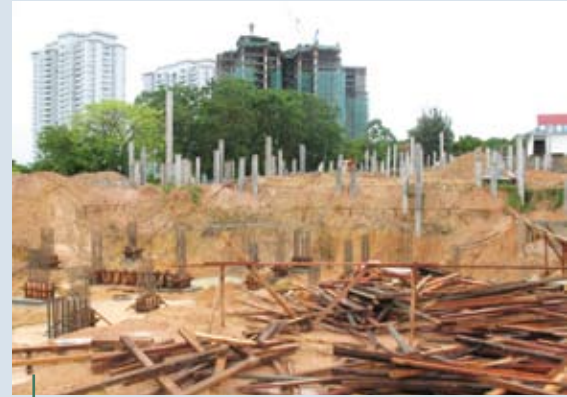
Construction of teachers' training college in Penang.
