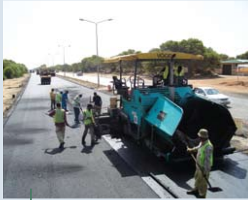
Road rehabilitation works in Libya.
