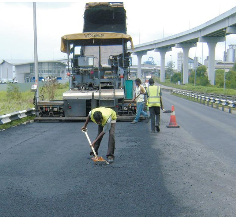
Cold-In-Place Recycling (CIPR) Works at Pulau Indah, Klang.
