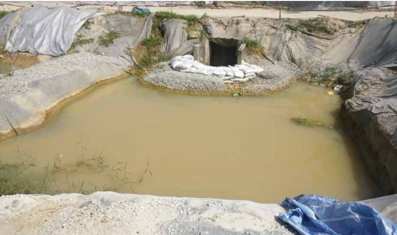
Maintenance of Silt Trap as Part of Erosion and Sediment Control Plan
