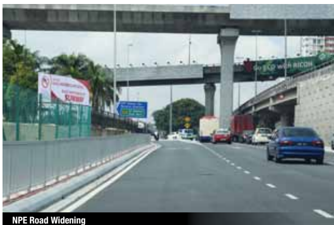
NPE Road Widening
