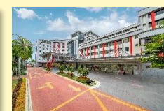
Sunway Medical Centre (Tower A & B)
